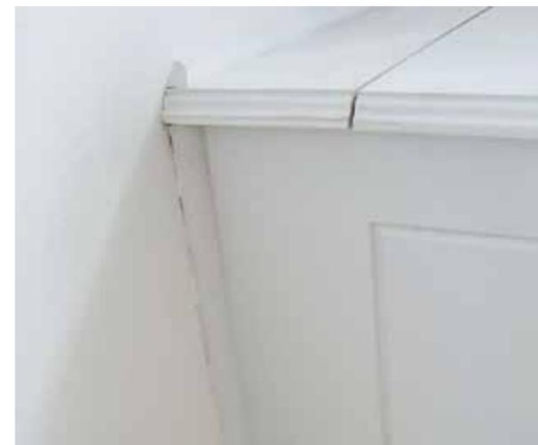
**9** Prime and paint the exterior surfaces using a spray technique to ensure a smooth, Duco-style finish. While using a spray gun inside, take any necessary safety precautions and ensure sufficient ventilation in the room. There is no need to paint the inside of the window seat as this will not be visible when it is closed. However, you can if you want to.
